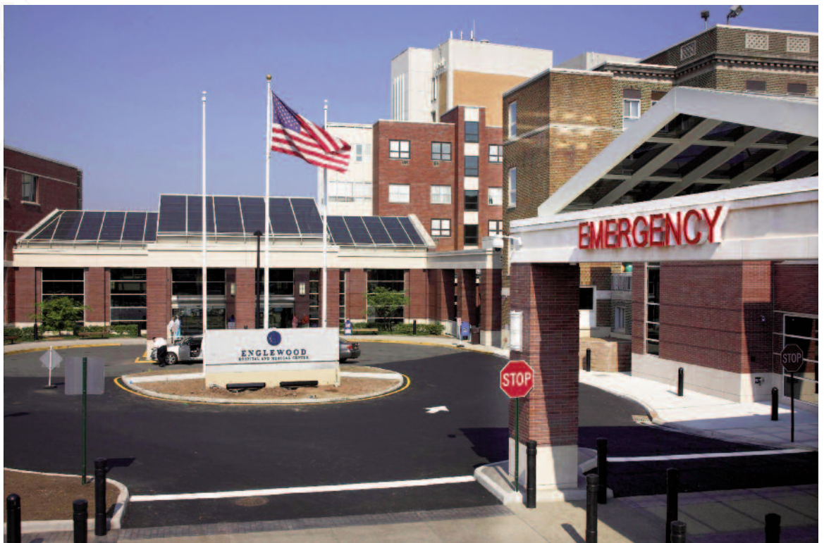
Englewood Hospital and Medical Center
