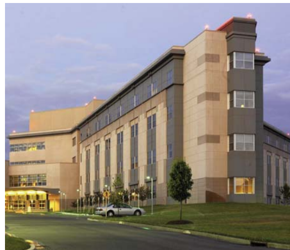
South Jersey Regional Medical Center ext.
